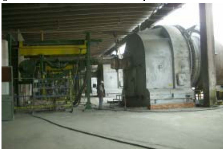
Figure 5.3.2 – Blended Waste Feed System at Cement Kiln
