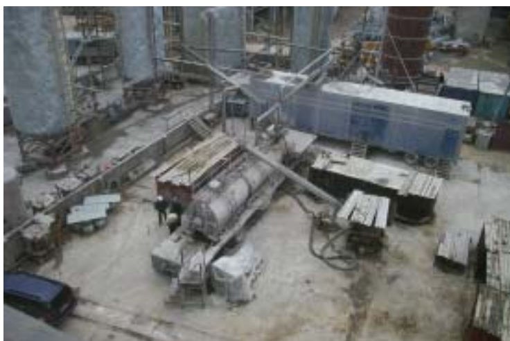
Figure 5.3.1 – Sotem Organic Waste Blending Facility
